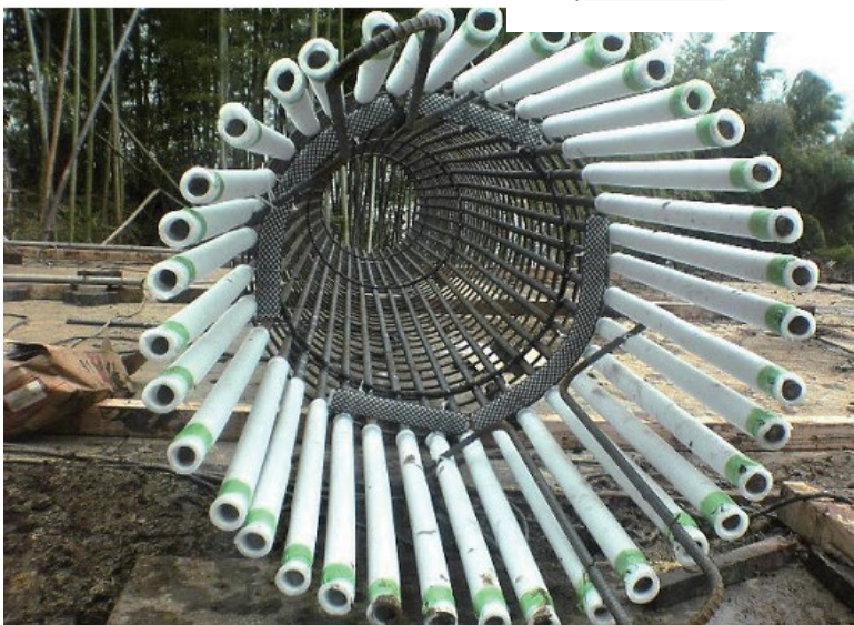
Installation of QUI CUTTER and Debonding Foam
