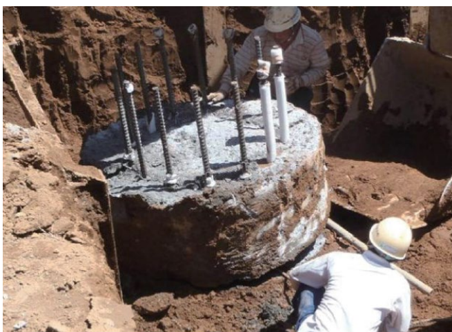
Lift off the 1 st stage of pile head concrete
