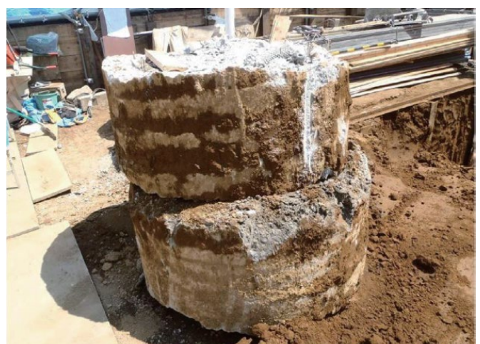
Removed pile head concrete
