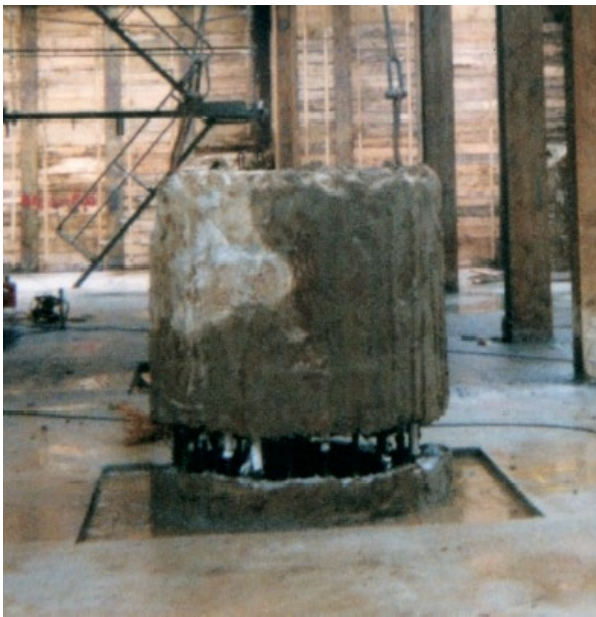
Lift off the pile head concrete
