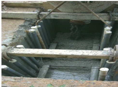
Lowering setup into trench
