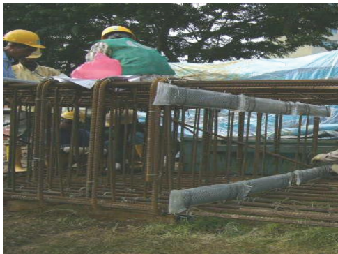
Installation of Qui Cutters
