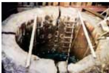
Demolition of Pillar
