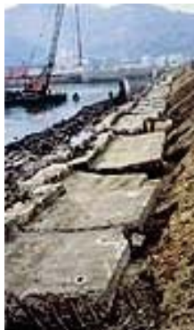
Demolition of Retaining Wall
