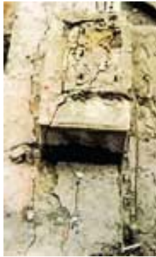
Demolition of Concrete Foundation for machinery
