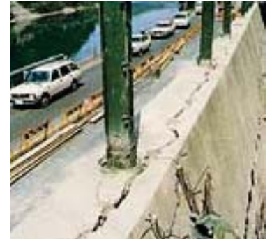
Demolition of Retaining Wall
