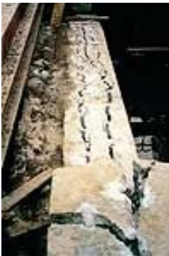
Demolition of Temporary Concrete Structure
