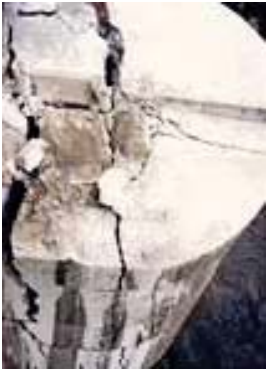
Demolition of Pier
