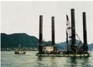
Demolition under Water
