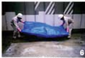
Covering with a plastic sheet
